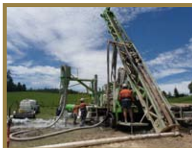
Right: Diamond core drilling
