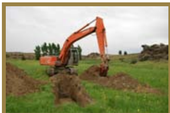
Bulk testing underway within the Manuherikia Valley, Central Otago
